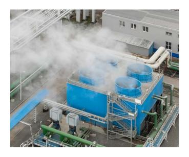
In fact, they use the natural law according to which the forced evaporation of a minimum quantity of water causes a lowering of the temperature of the main fluid mass.
